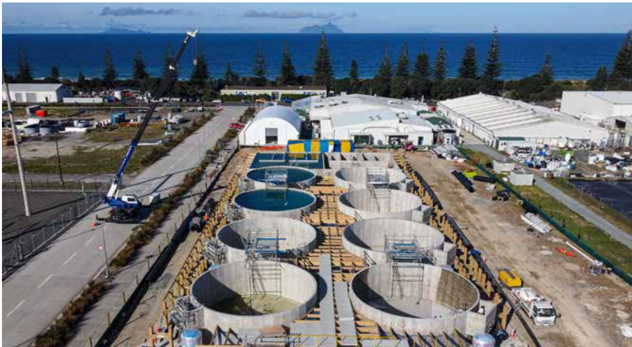
The Northland Aquaculture Centre at Bream Bay. The tanks at an early stage of construction. The whole facility is completely covered in – ready for the production of 600 tonnes of Haku kingfish a year. Image: CB Civil.
