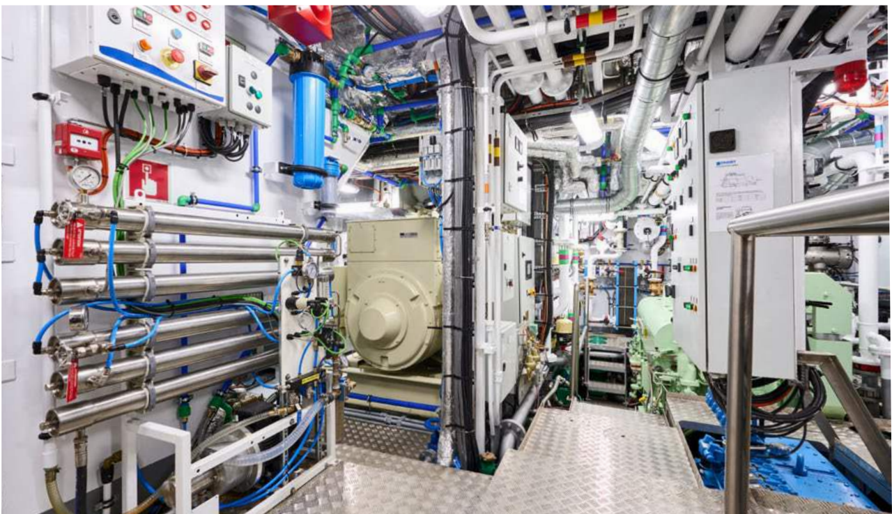
Kaharoa II 's engine room. The vessel is supported by systems enabling it to operate as sustainably as possible, while maintaining the ability to adopt new renewable-low carbon energy technologies.
